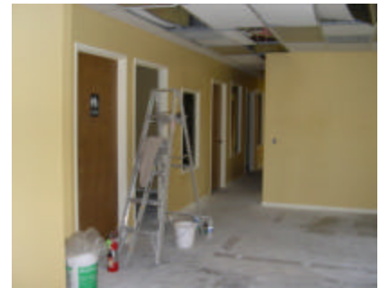
With old carpeting removed, painting had begun.
